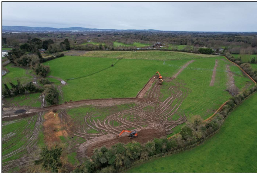
Plate 1 Aerial view of Phase 1 topsoil stripping, looking south
