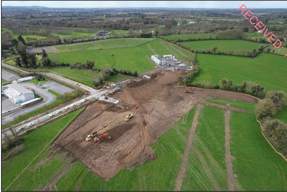
Plate 7 Aerial view of topsoil stripping north--east of compound, looking south-west
