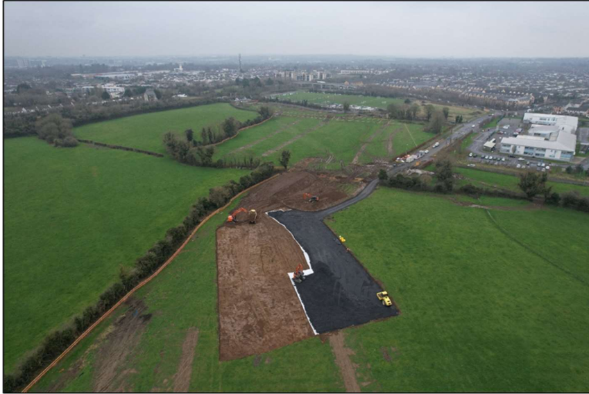
Plate 4 Phase 1 topsoil stripping completed, looking north
